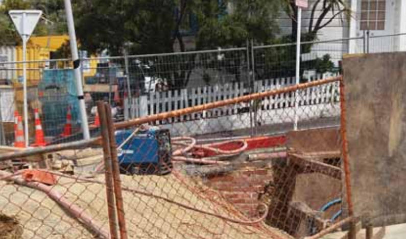
A brick sump was found beneath Hargreaves Street. It is a stand-alone stepped structure, and is well-preserved after being underground for around 100 years. In its day, Mt Cook was Wellington's brick-production area, with one of its brick factories (Hill's, later Hutson's) having formerly been just across the road on the Housing NZ apartment site between Hargreaves and Rolleston Streets.
